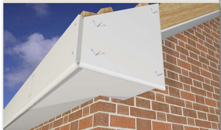
Fig. 26. Magnum Roundnose Fascia box end with vertical cut junction.
